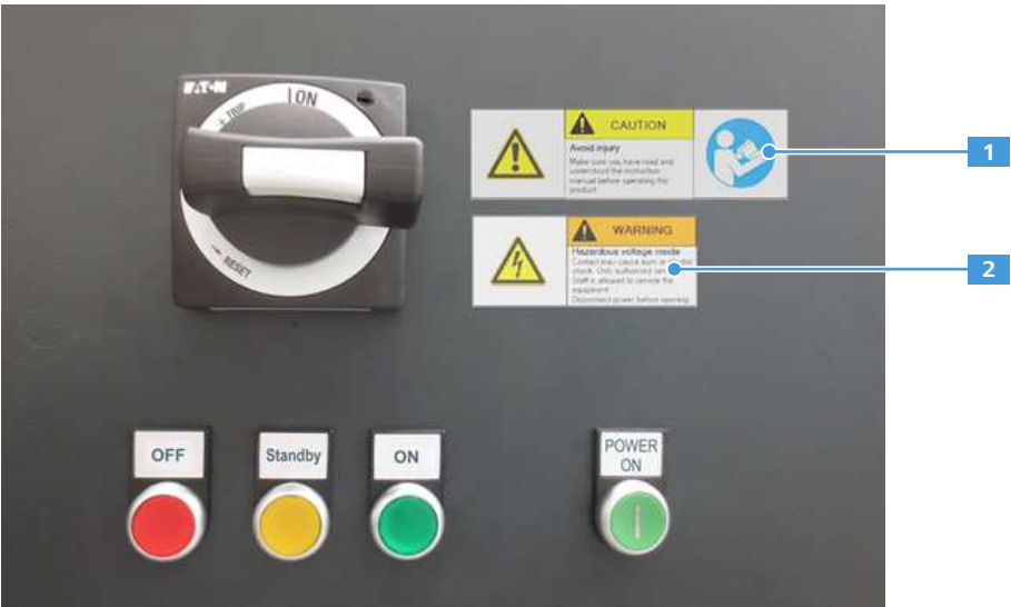
Fig. 2.8: Safety labels at the main switch area
